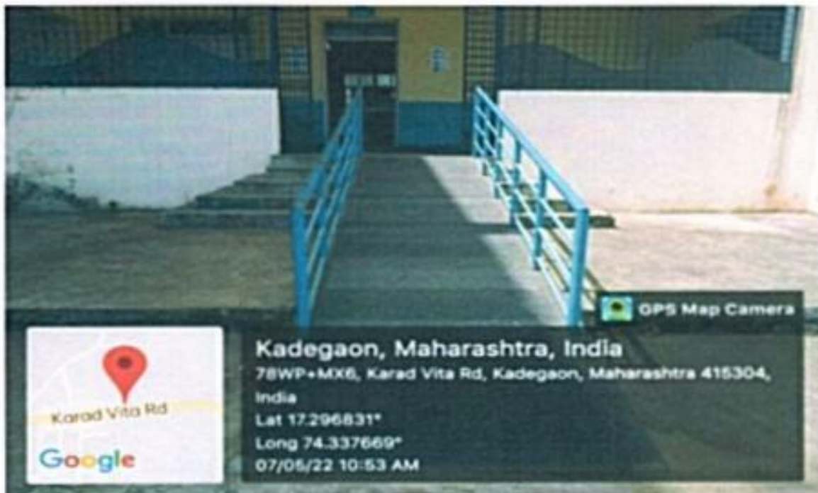
Ramp for easy access to classroom
