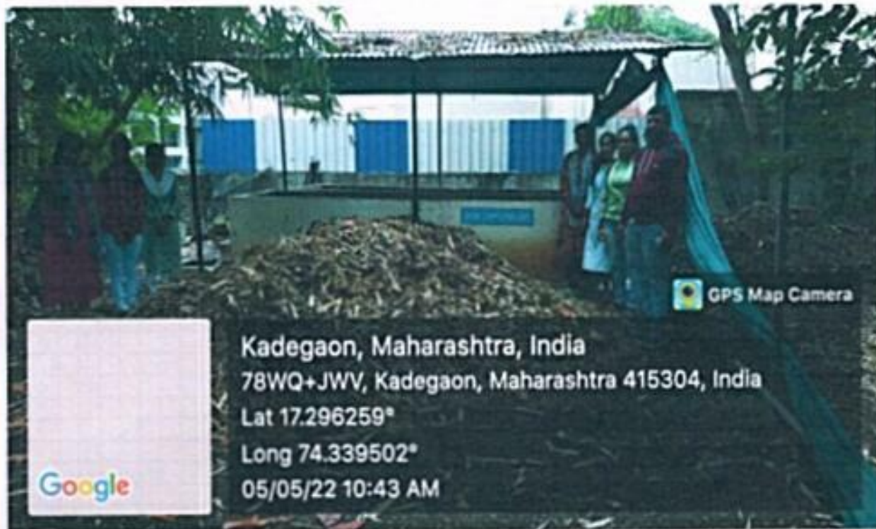
Vermi composting Unit in college Campus
